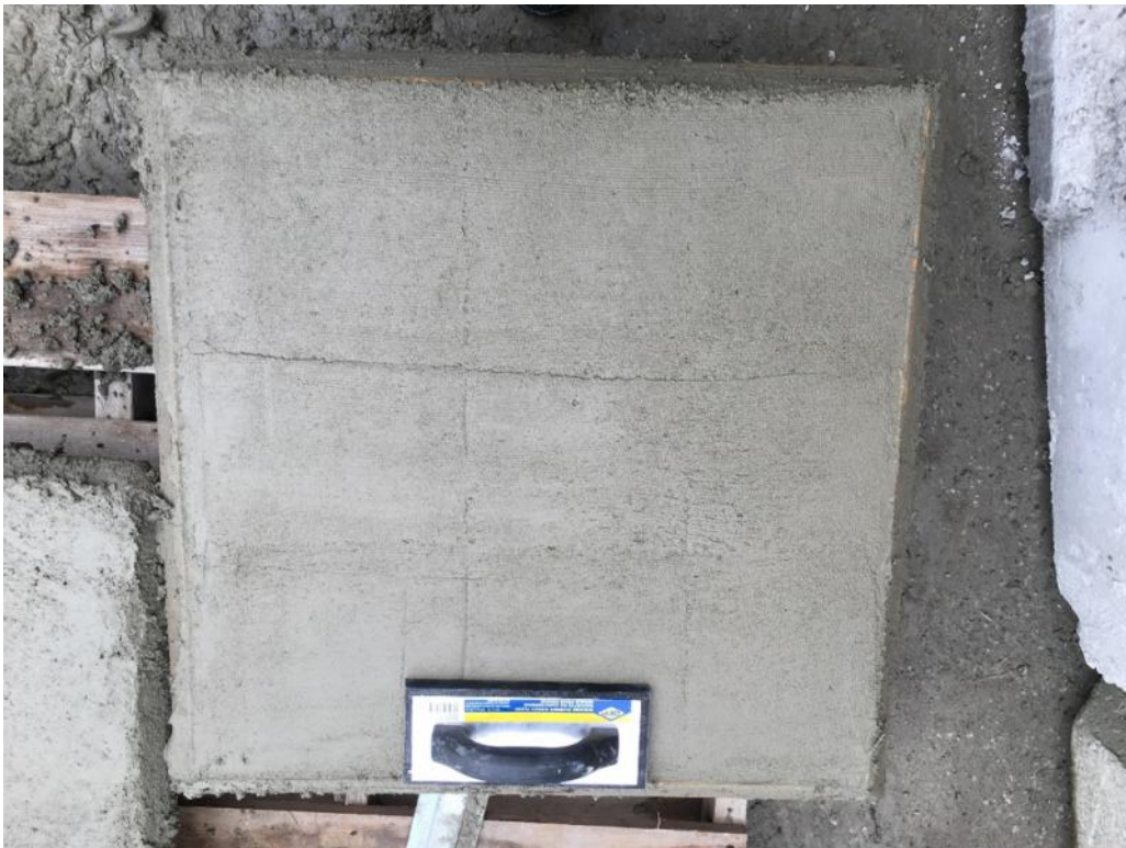
Figure E-6: Plain wet-mix shotcrete mix finish: textured rubber float finish
