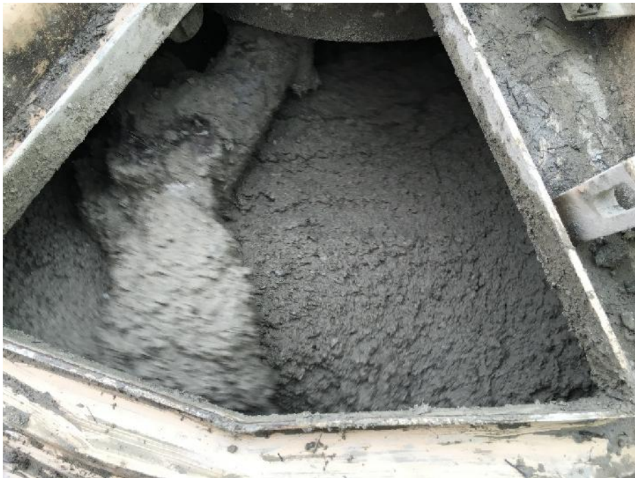
Figure B-2: Wet-mix shotcrete inside the pan mixer
