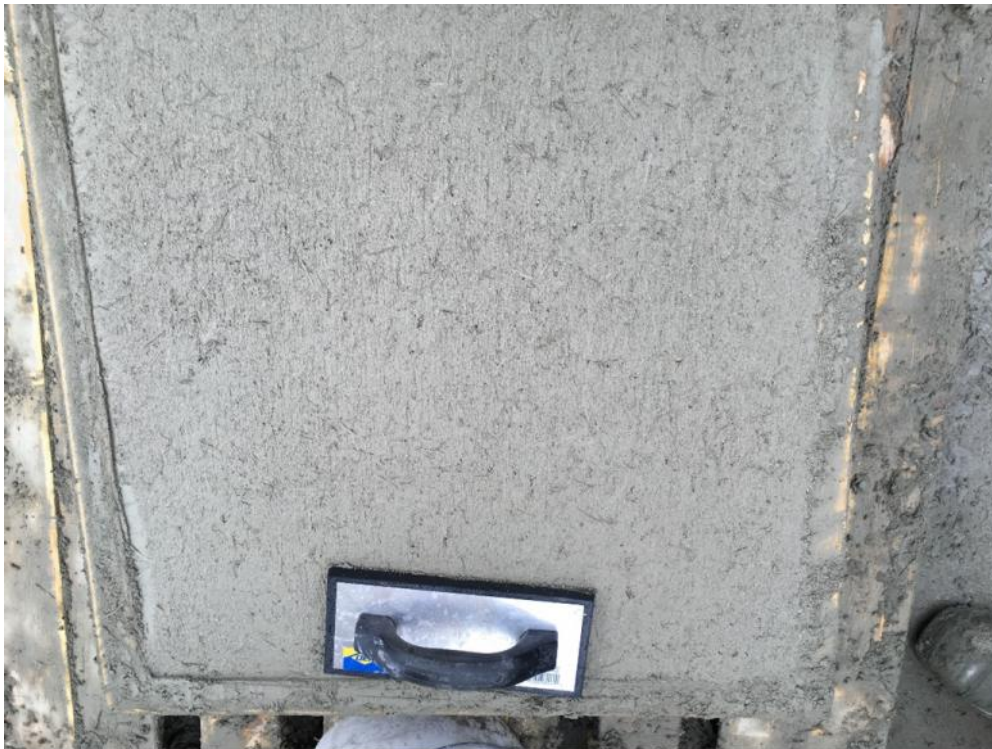
Figure E-12: Microsynthetic fiber mix finish: textured rubber float finish
