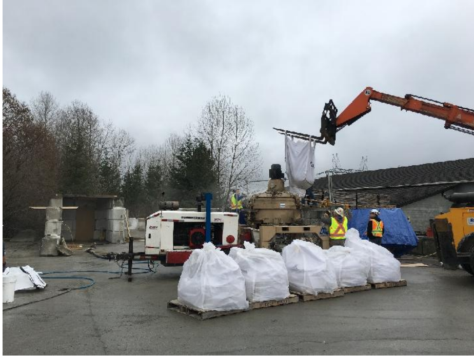
Figure B-1: Pre-bagged materials (0.5 yd 3 ) discharged into the panel mixer, water and water reducing admixture manually added to adjust slump. Putzmeister wet-mix shotcrete pump used to pump the shotcrete.
