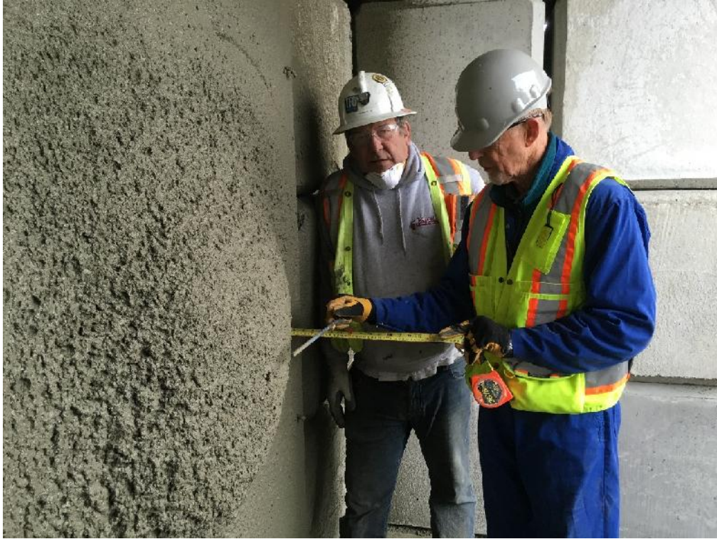
Figure B-7: NForce-Fiber wet-mix shotcrete vertical thickness build-up & measurement
