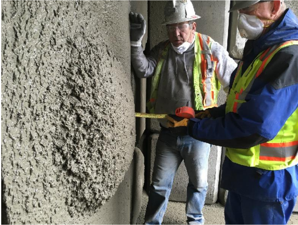
Figure B-8: Measuring the vertical thickness build-up of dry-mix shotcrete
