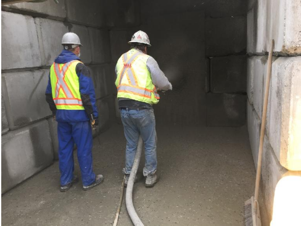
Figure B-6: Shooting vertical build-up
