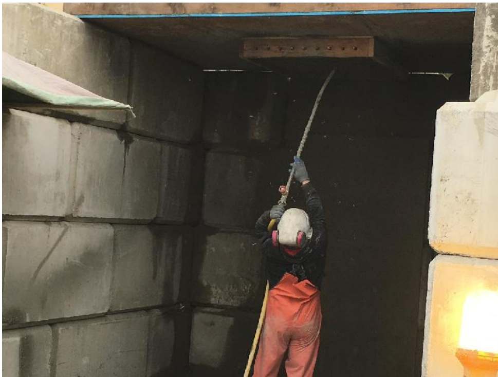
Figure B-21: Cleaning overhead rebound panel after each shoot
