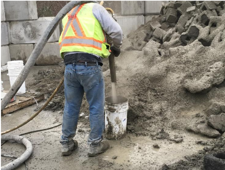
Fig. B-19, Shooting into bucket to test as-shot air content
