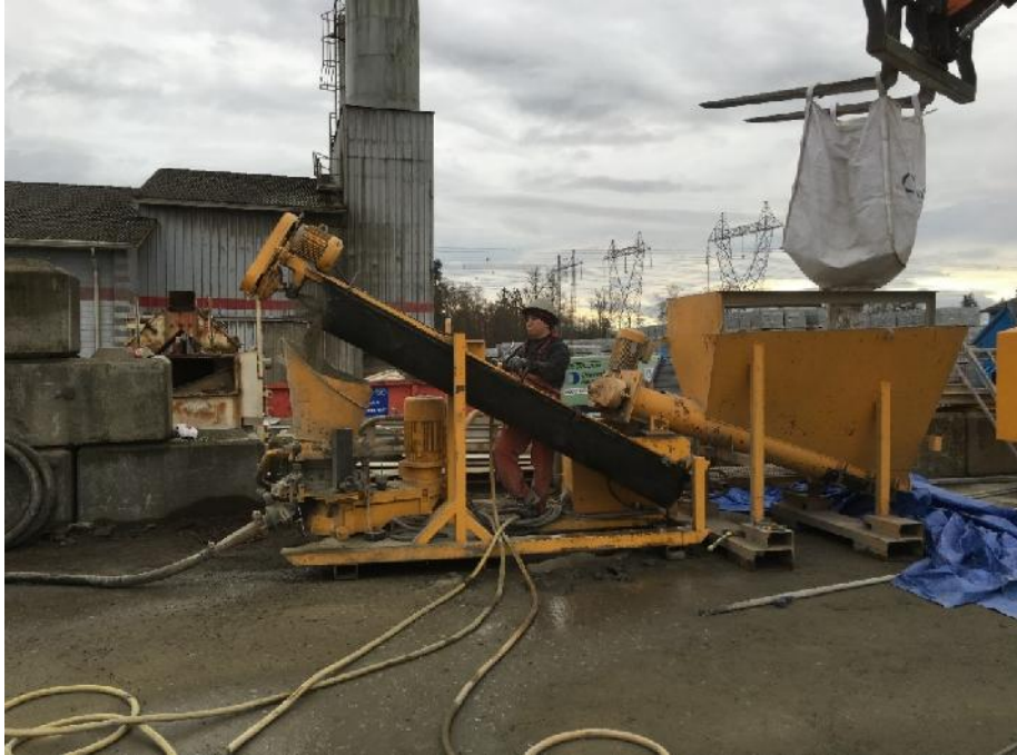
Figure B-1: Pre-bagged materials (0.5 yd 3 ) discharged into the hopper, then discharged by an auger into the predampener: water added to predampen the materials to moisture content of 4-6%, and materials discharged into an Aliva rotary gun.
