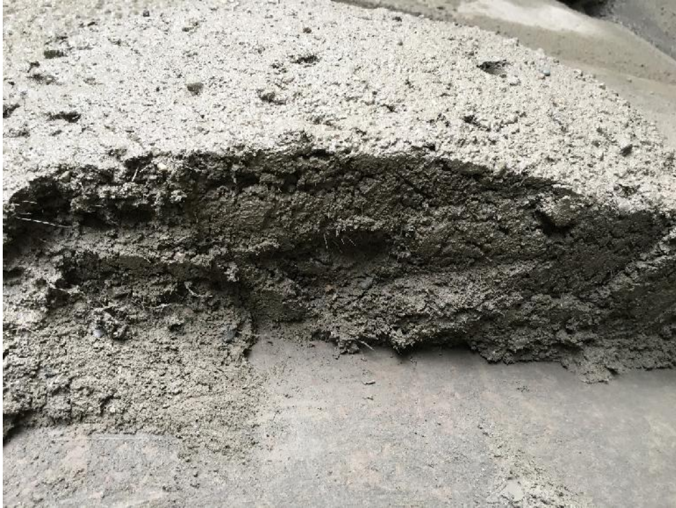
Figure B-10, Cutting off the vertical dry-mix shotcrete build-up
