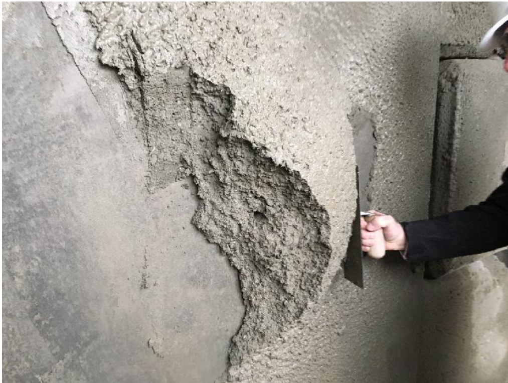
Figure B-9: Cutting off the vertical dry-mix shotcrete build-up
