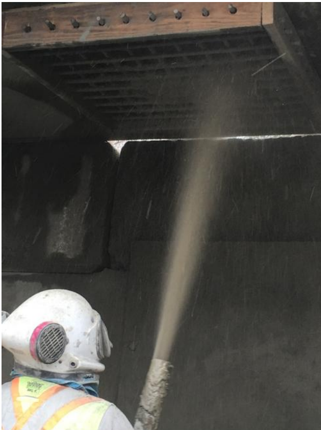
Figure B-17: Shooting overhead rebound test
