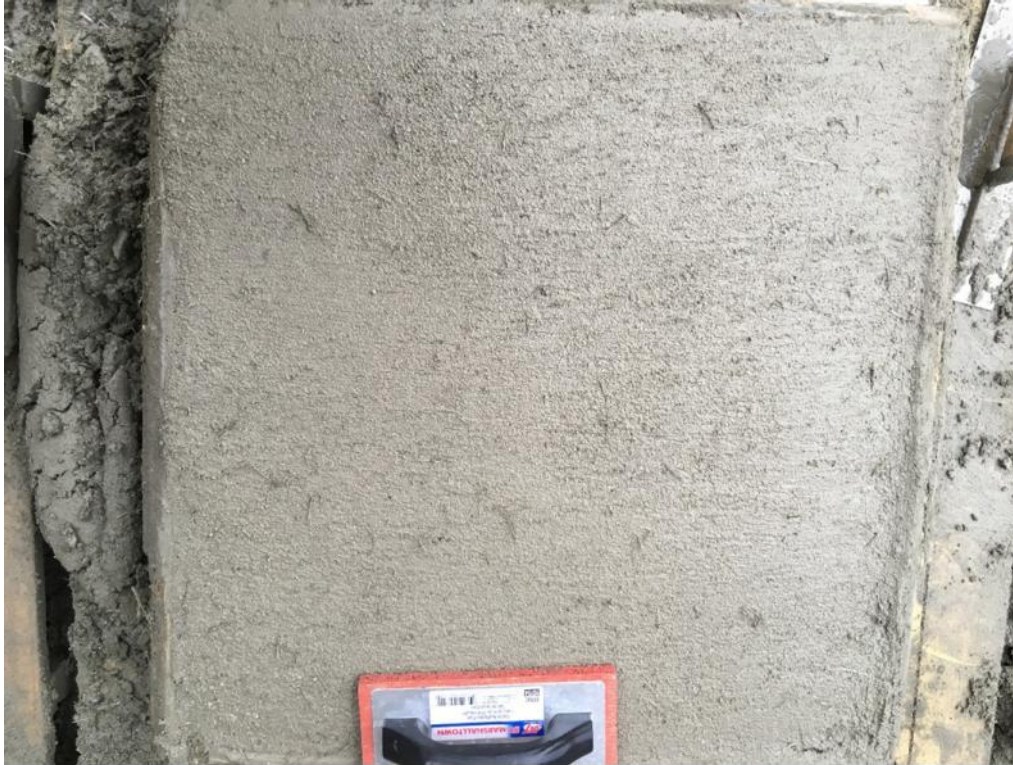
Figure E-13: Microsynthetic fiber dry-mix shotcrete finish: sponge float finish
