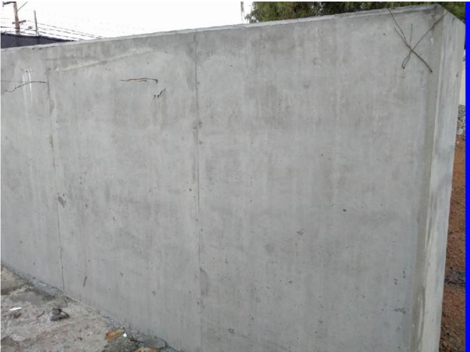
Fig.11 Stripped face of L-shaped wall
