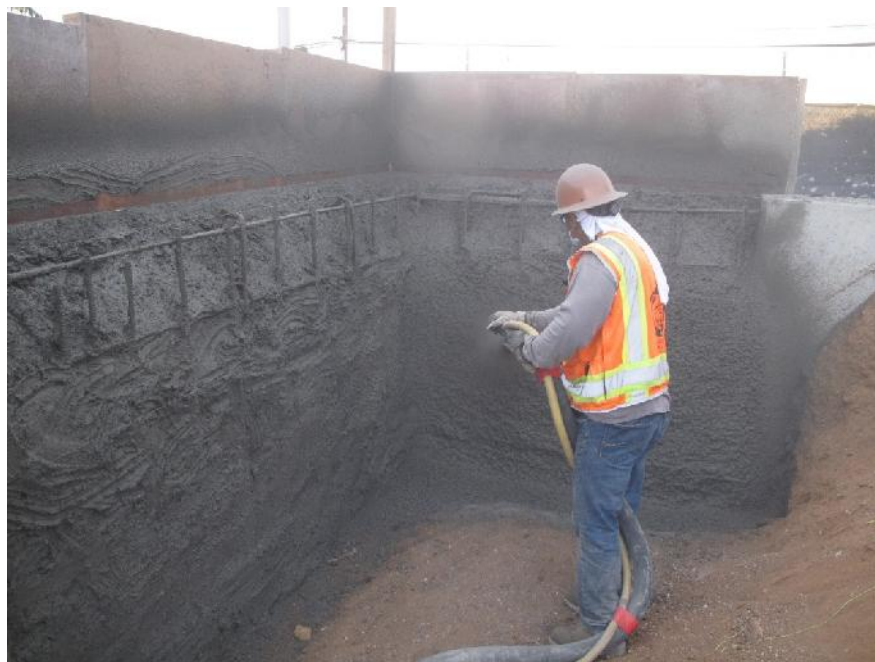
Fig.7 Shotcrete application on L-shaped wall
