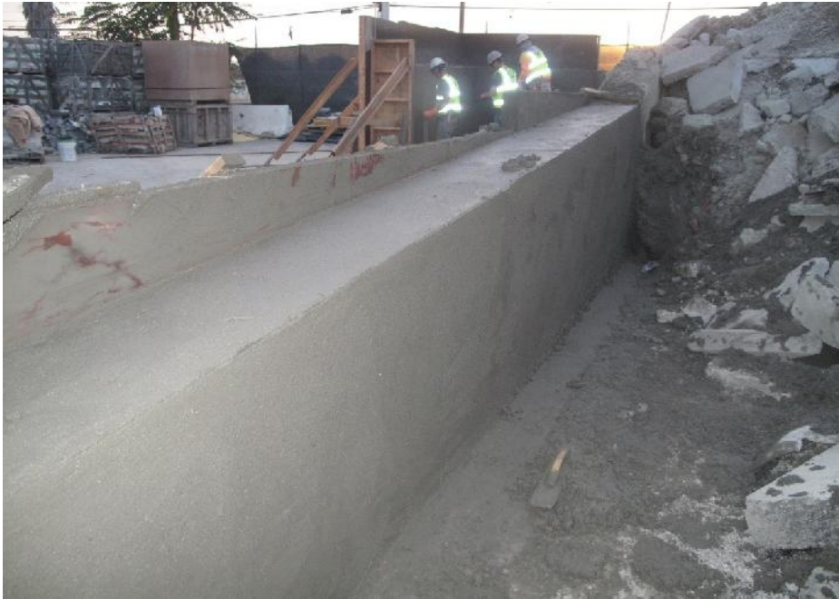
Fig.10 View of finished straight wall
