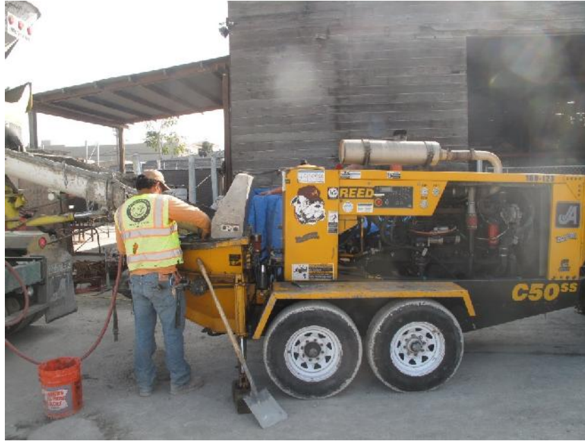
Fig.3 Reed C50 pump used to pump shotcrete
