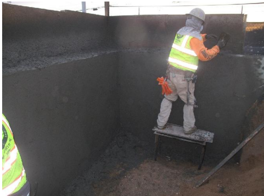
Fig. 9 Finishing of L-Shaped Wall
