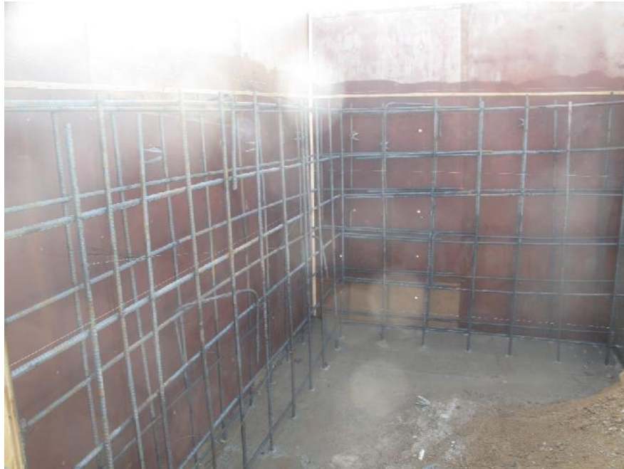
Fig.5 Formwork and rebar for L-shaped shotcrete wall
