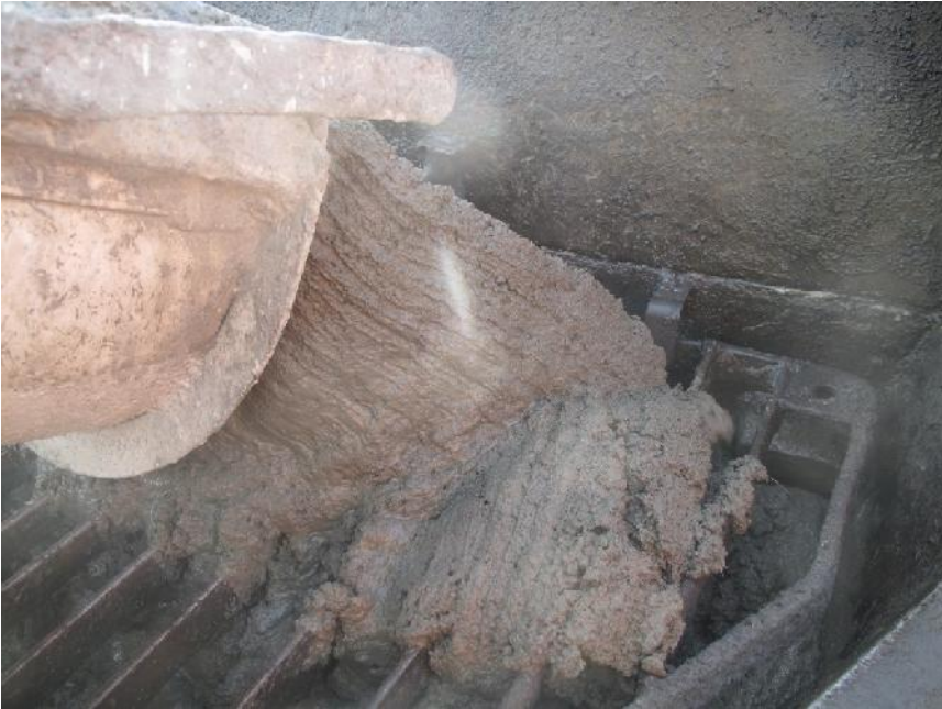
Fig.2 Discharge of fiber-reinforced shotcrete into pump hopper
