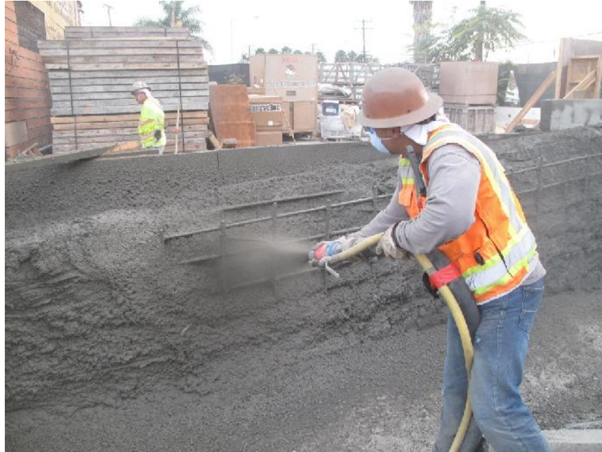
Fig.6 Shotcrete application on straight wall
